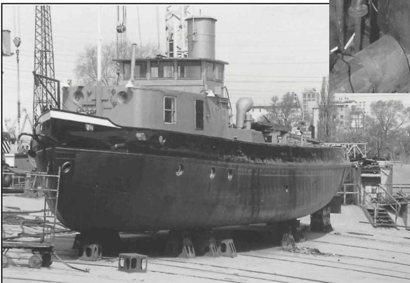
Renovation works in the Wroclaw River Shipyard.
