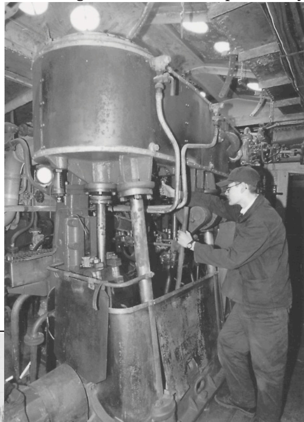
Inside the engine room on "Nadbór"
